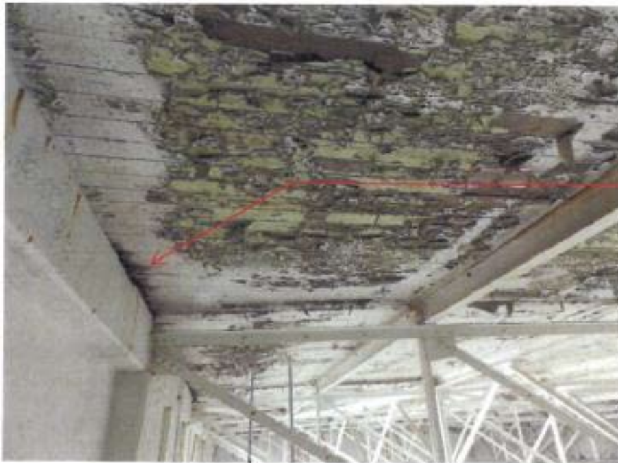
Example of Structural Deficiency Due to Dry Rot
